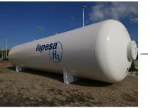
Buffer Tank 50 m³; D:2450 L:11510 10-40 bar 180kg
